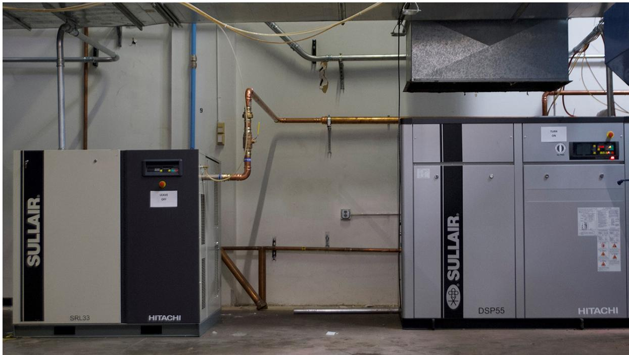
One of the most challenging parts of installing a new compressed air system can be correctly sizing it for both today and years for now—all while maintaining optimal efficiency. Choosing the wrong air compressor(s) for your facility can significantly increase costs due to wasted energy or even production problems.
