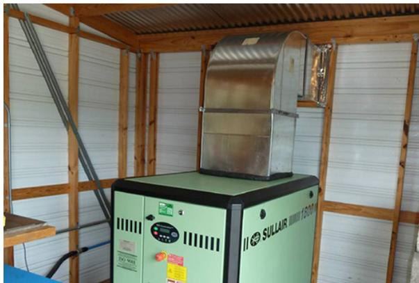
Additionally, you do not want to install an industrial air compressor in an area with a high amount of particulate. That can clog a cooler and cause overheating.
