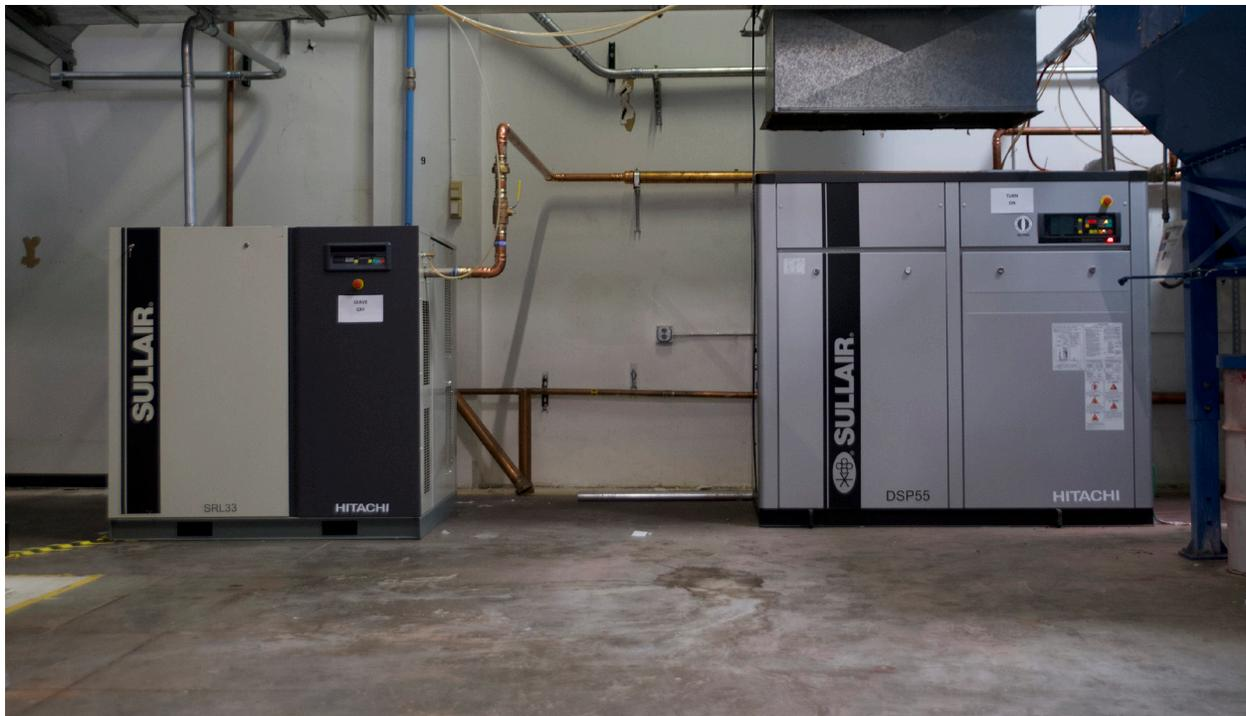
The most expensive component in the total cost of compressed air is energy. Over the lifespan of a typical compressor, energy often costs several times more than the purchase price of the compressor. According to the U.S. Department of Energy, electricity represents more than 75%<sup>1</sup> of the total costs of an air compressor over its lifecycle.
