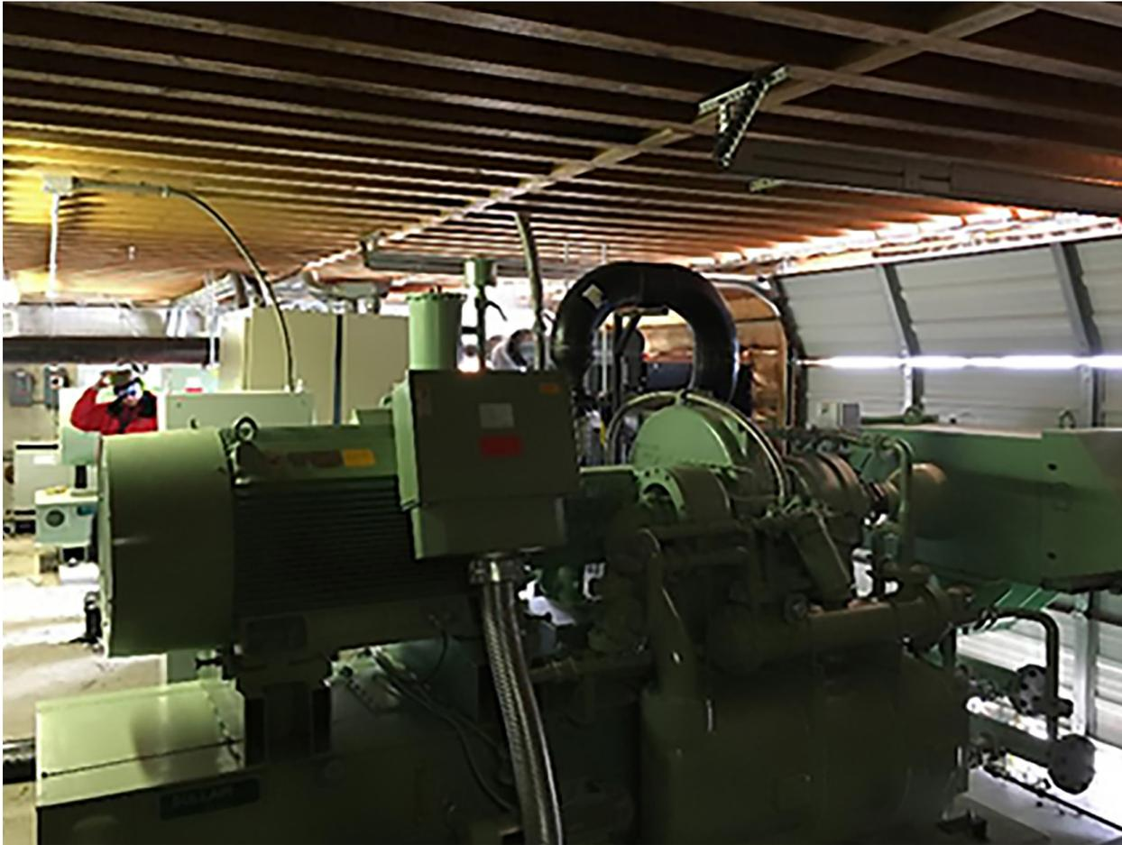
*One ski resort's compressed air system consists of two Sullair TRA 600 hp centrifugal compressors*
