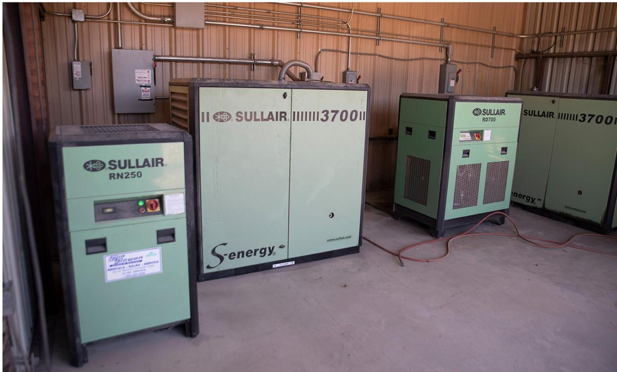
high ambient temperature because it raises the inlet air temperature (see above), refrigerated dryers are also affected more directly. As the ambient air temperature increases, the refrigerated dryer dissipates heat less effectively, which makes the cooling process less efficient, leading to a reduced dryer capacity.
